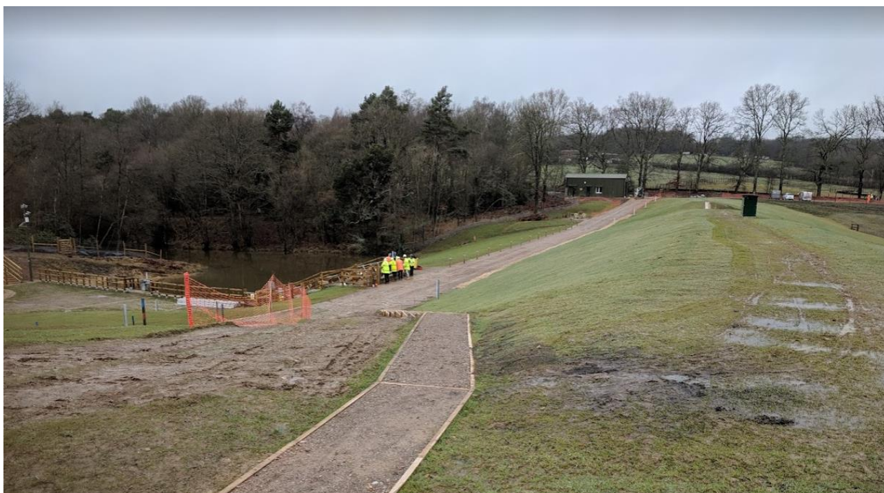
Clays Lake project completion hand-over in 2019
