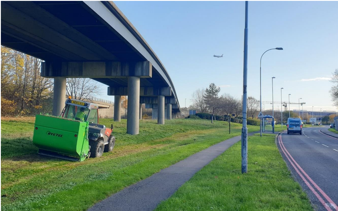
Glendale Services road verge cut and collect © Rachel Bicker
